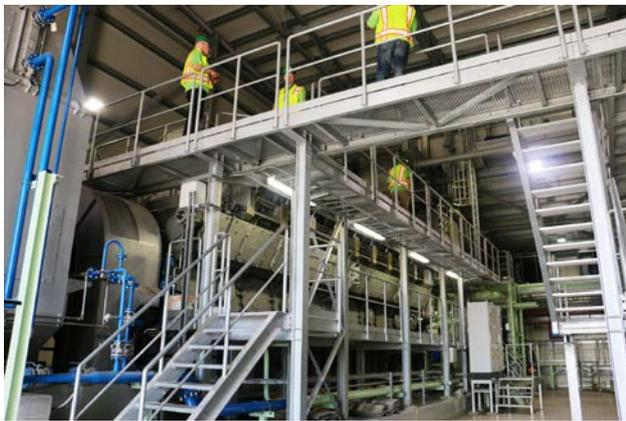
*One of the two 18.5MW MAN 48/60 engines in Engine Room 6, the newest phase of the Caribbean Utilities Company power plant in Grand Cayman.*
