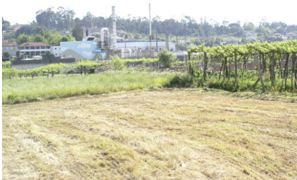
The TMG SPE industrial cogeneration plant at Vila Nova de Famalicão in Portugal feeds electrical power to the grid and generates process steam for an adjacent textile works
