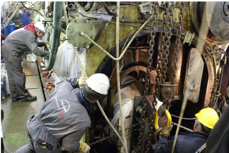
*The under-slung 6L58/64 crankshaft is hoisted back in place*
